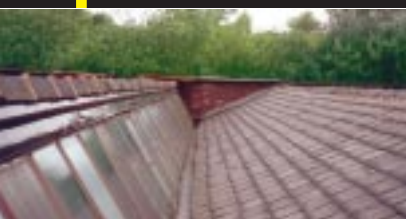
Re-lined north light roof gutter
