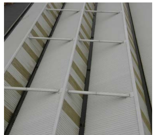
Gutters in excess of 200m have been successfully lined with Gutterline
